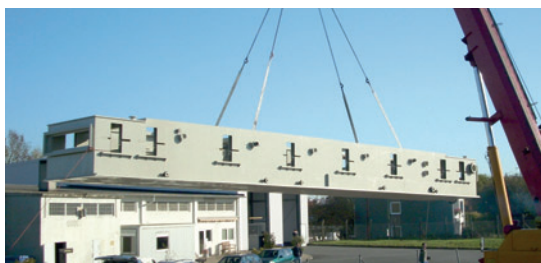
Delivery of the pickling tanks to the Rasselstein steel plant
